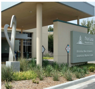
Entrance to Nor-Lea Hospital
